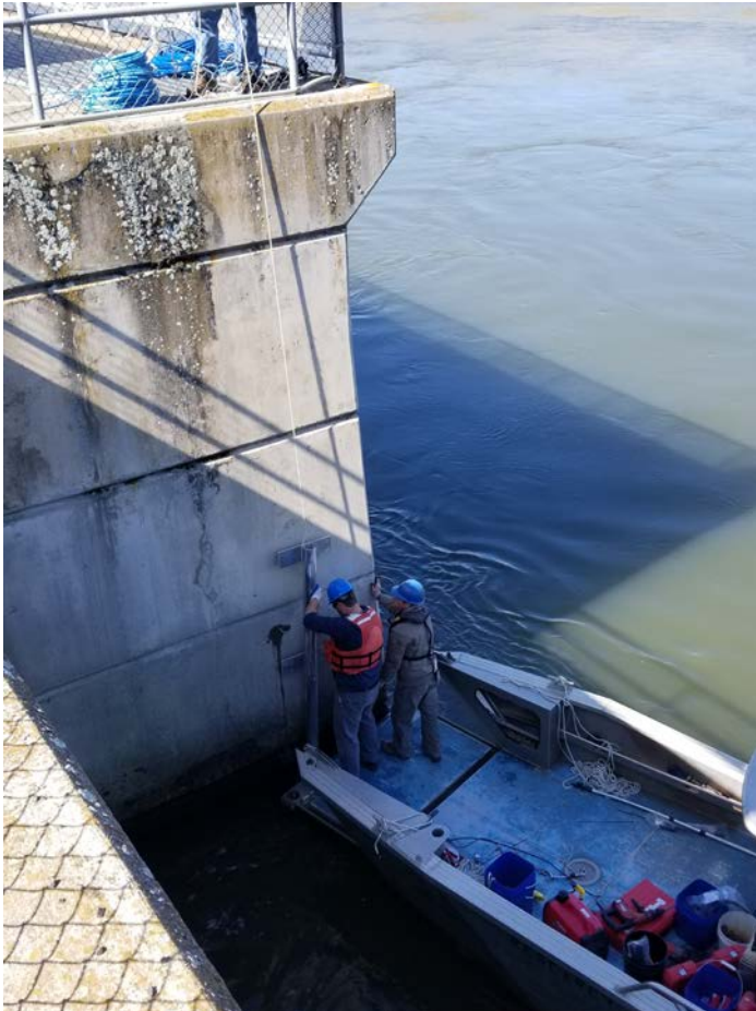
Installing trolley pipes near the navigation lock discharge.
