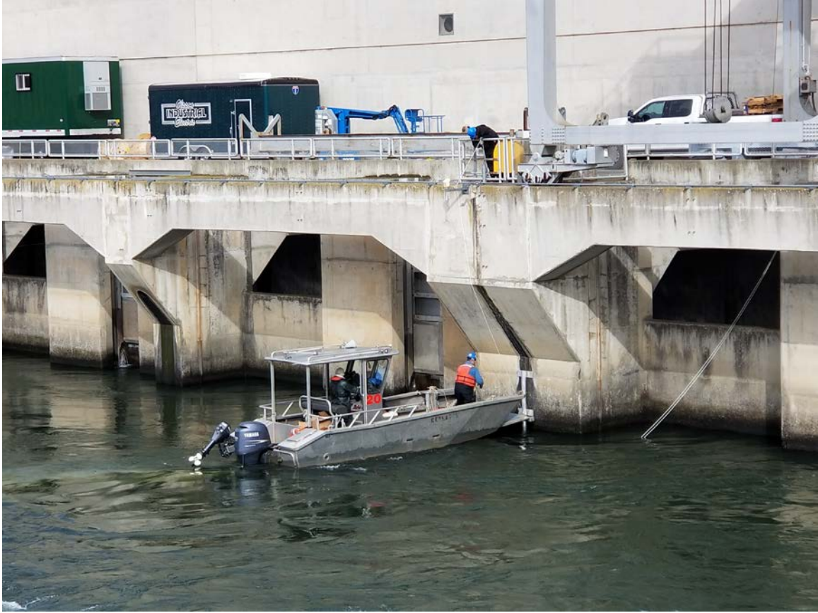
Installing hydrophone trolley pipe, powerhouse.
